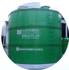
Biogas plant 1 Tonne Capacity
